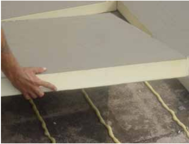
DERBIBOND PG - Pump Grade Insulation Adhesive eliminates the need for mechanical fasteners
